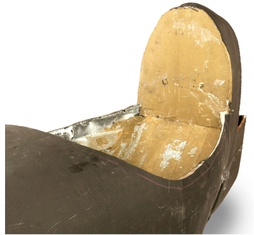
Figure 3: Smooth interior surface of bulkhead and front cavity.
